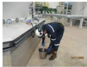
3. Connect bonding (sampling and blanket)
